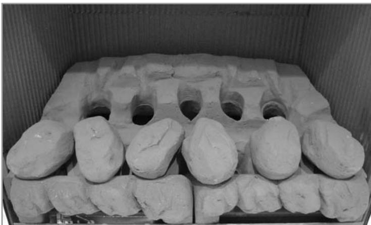
4. Open the bag of 16 moulded coals. All of the coals are the same. Take six coals and place them as shown. Care should be taken to ensure that the coals bridge the gap between the front coal and the four coal supports at the front of the matrix.
