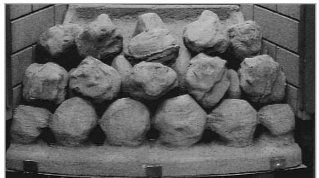
4. Take five more moulded coals and position as shown to form the 'second row' of the fuel effect. The coals may be rotated as desired to fit into the gaps between the coal supports in order to create a random, realistic effect. Again, remember not to push the coals down too far into the valleys between the coal supports as this can have a detrimental effect to the flame picture.
