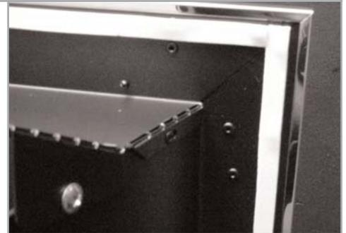
**CABLE FIXING.** For fixing of the fire by the cable method, see the relevant section. The cable fixing locations should be marked on the back of the opening and the holes drilled. Fit the wallplugs and eyebolts to these holes.
